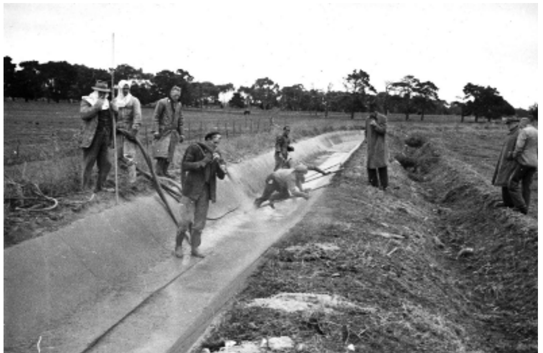
▲ Figure 15. Gunite lining of the 1K channel, Werribee District, c. 1953-54 Source: Victoria. State Rivers and Water Supply Commission, rw008097, Rural Water Corporation collection. Werribee, State Library of Victoria
