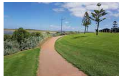
4 EXISTING STEEP PATH SECTION TO BE REGRADED AND REPLACED WITH 2.5m RC SECTION
