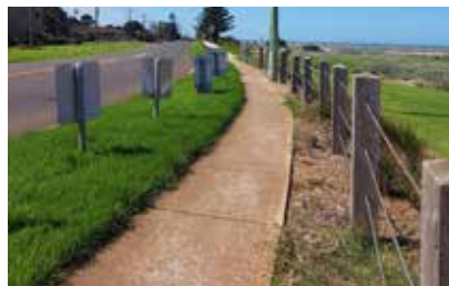
1 1 - 1.5m WIDE EXISTING PATH SECTION TO BE WIDENED TO 2.5m ON DECK SECTION
