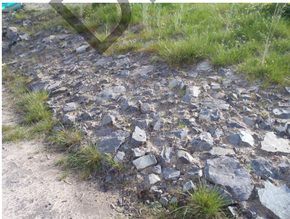
Photo 1: Melbourne Water accepted Type 5 rock beaching
