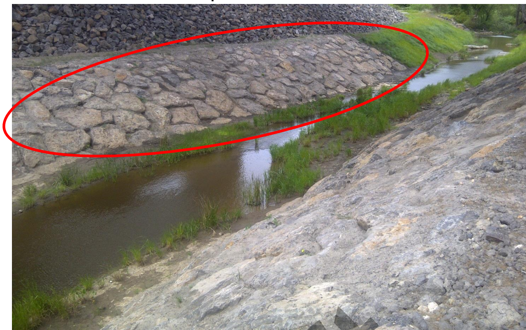
Photo 2: Melbourne Water accepted Armour Stone
