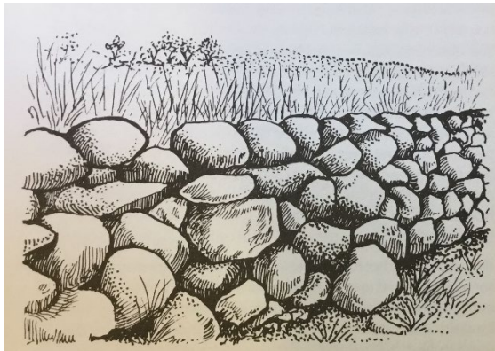
Figure 11. Drystone walling on the Western Plains. (Source: Winty Calder, Beyond the View , 1981, p. 97)
