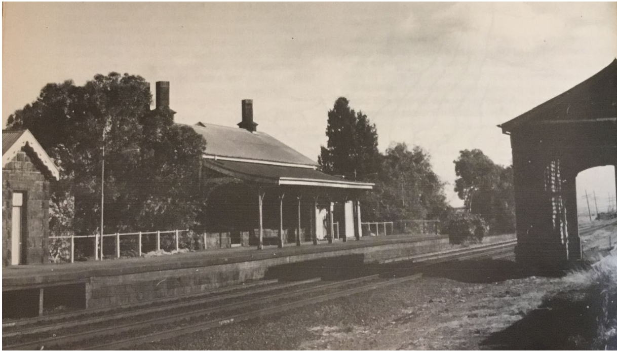
Figure 22. Bluestone railway station and engine shed at Little River, constructed in 1864. (Source: Winty Calder 1981, Beyond the View )
